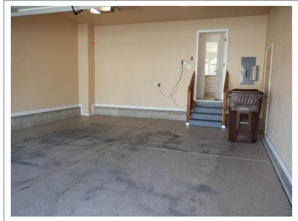
Figure 10.2 - Overview of garage area.
