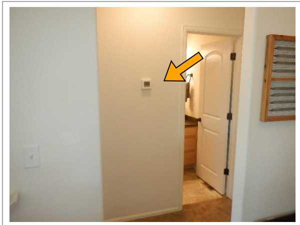
Figure 4.1 – Location of heating thermostat at main floor living area
