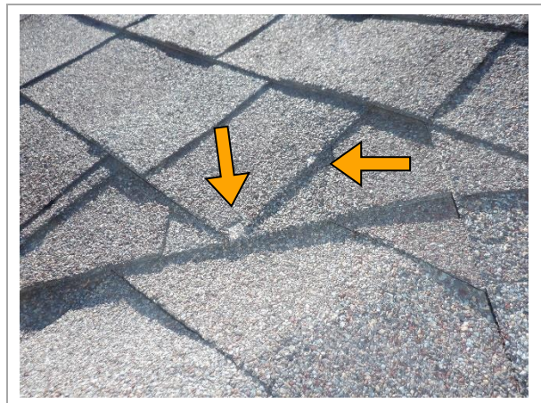
Figure 1.4 - Example instance minor shingle damage.
