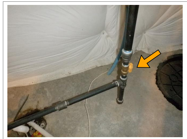
Figure 6.6 – Presence of gas shutoff valve verified at water heater
