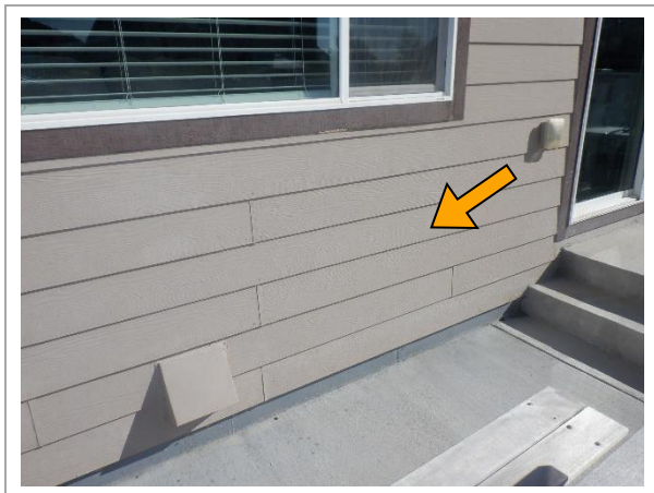
Figure 2.3 – Example area paint fading/chalking.
