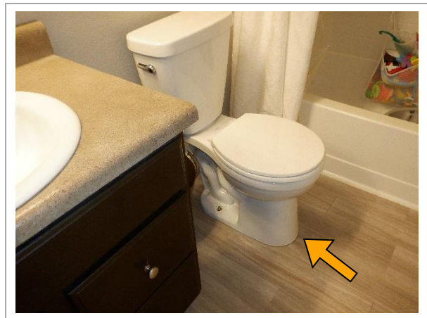
Figure 6.10 - Loose toilet base at main floor bathroom.
