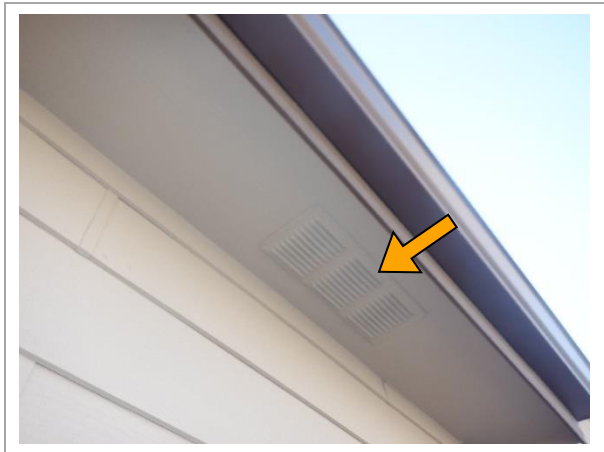
Figure 9.2 – Attic ventilation – soffit vents
