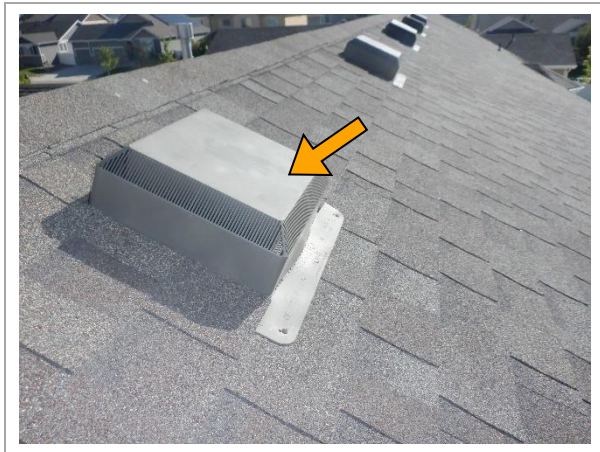
Figure 9.1 – Attic ventilation – ridge/box vents
