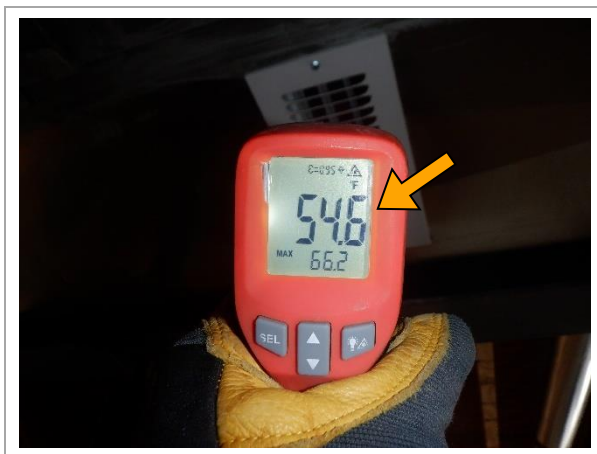
Figure 5.5 - Observed AC outlet temperature
