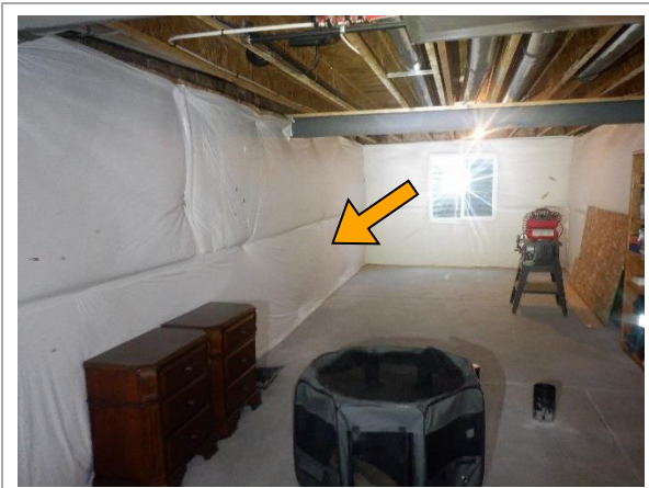
Figure 3.3 – Insulated foundation walls in basement area.
